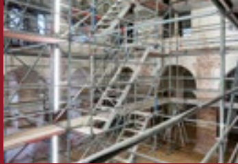
Baufortschritte in Corvey
